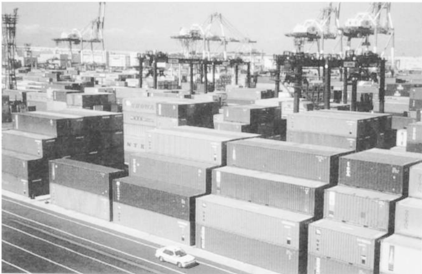
Figure 2.3 Container port, Yokohama, Japan.
