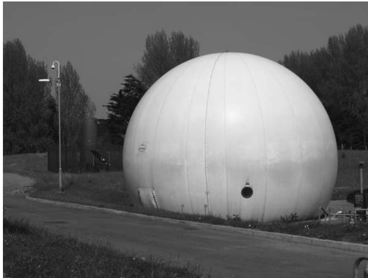
FIGURE 19.7 Gas storage bag with gas flare in the background where excess gas is burnt to prevent methane, which is a greenhouse gas, escaping to the atmosphere.
