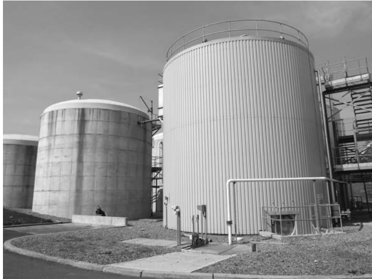
FIGURE 19.6 Two stage anaerobic digestion with heated mesophilic digester on the right and unheated settlement stage on the left. Excess supernatant (sludge liquor) is stored in the smaller tank on the extreme left prior to being returned to the inlet for treatment.
