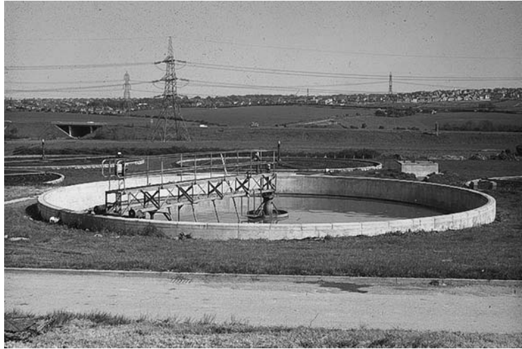
FIGURE 14.7 Radial flow sedimentation tank.
