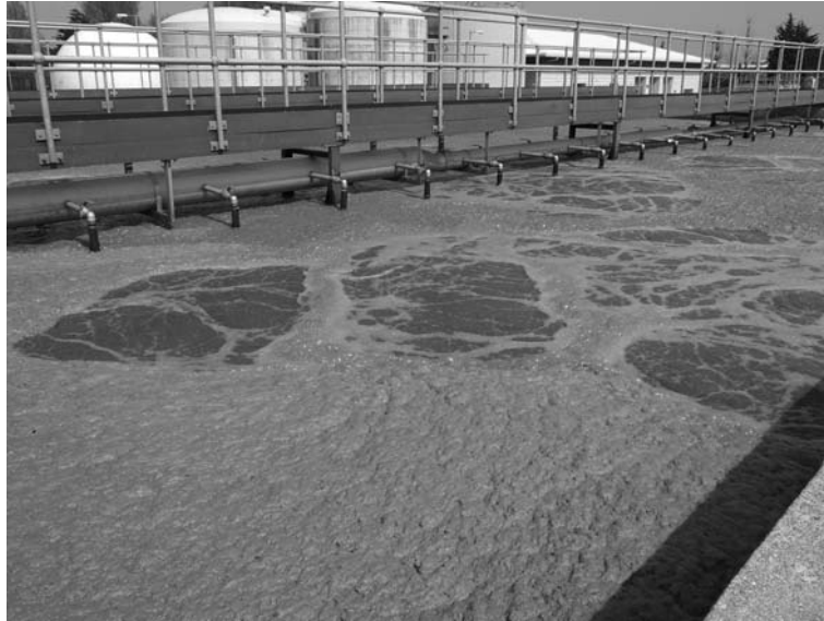
FIGURE 17.26 Diffused aeration activated sludge with Nocardia foaming.
