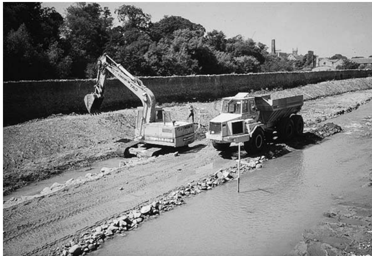
FIGURE 6.6 Flood prevention can cause significant damage to river ecosystems during construction. Wherever possible machinery should not be allowed in the water but should work from the bank or behind coffin dams.
