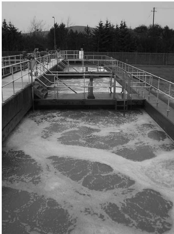
FIGURE 17.10 Plug-flow activated sludge made up of three separate cells aerated by air diffusion.
