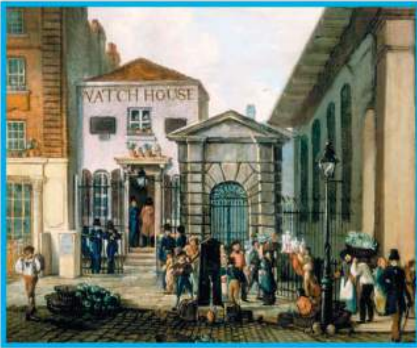
The Watch House in London's Covent Garden was built in 1729. In 1829, the newly formed Metropolitan Police took it over as headquarters of F Division, controlled by Superintendent Thomas.
